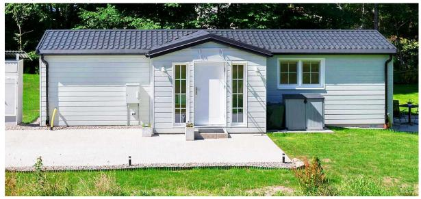
It was built with about 13 cm insulation with PUR foam in walls, ceiling and floor and triple insulating glazing. The façade is made of maintenance-free light grey Kerrafront Classic panels, which do not need to be painted and can be easily washed off with water. Inside, a floor with durable and stable MDF panels (Model Elton) was laid. On the walls and ceilings there are also MDF panels in white color, which makes the house look bright inside even in the dark winter.
